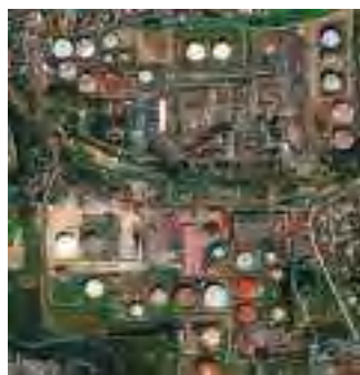
Kolonnawa Oil Tank Farm
