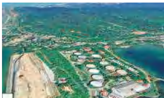
Trincomalee Oil Tank Farm
