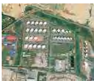
Muthurajawela Oil Tank Farm
