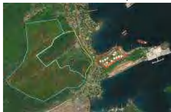
Trincomalee Tank farm Complex
