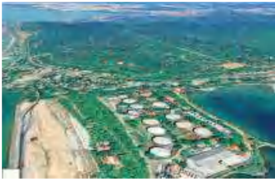
Trincomalee Tank farm Complex
