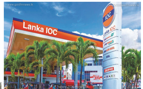
Lanka IOC Fuel Station
