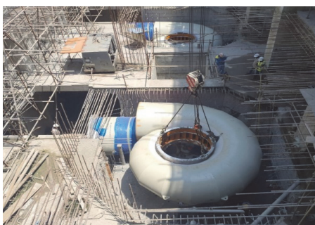
Powerhouse Spiral Casing Installation
