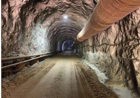
Head Race Tunnel Construction work
