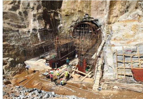
Diversion Tunnel Intake
