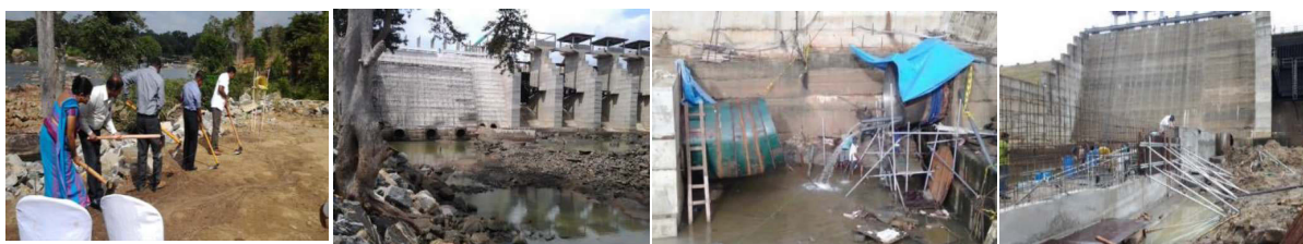
Initiating construction works
