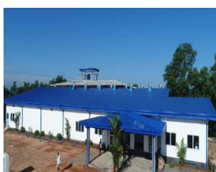
Factory Front view
