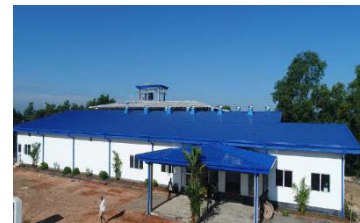
Factory Front view
