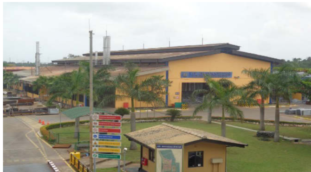
Sapugaskande Galvanizing Facility
